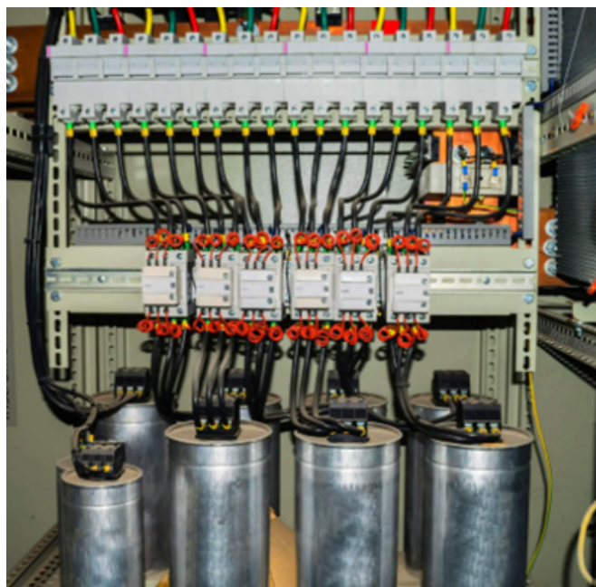
Figure 9: capacitor bank
