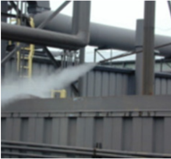
Figure 26: Steam leaks are a loss of condensate and energy - Left
